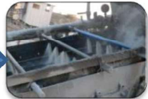
Washing & Sludge Removal
